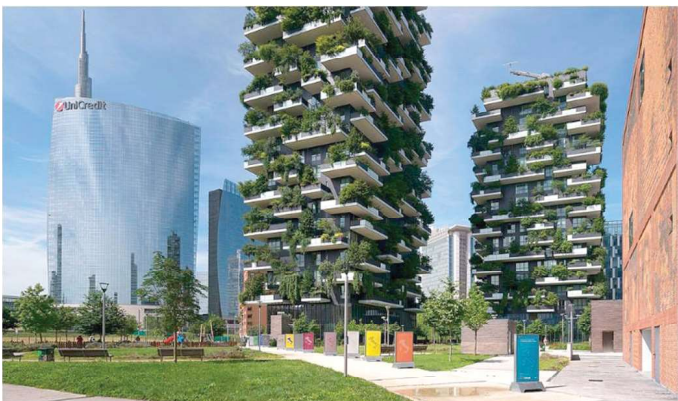
Fig.4. The Bosco Verticale, a residential tower [5]
